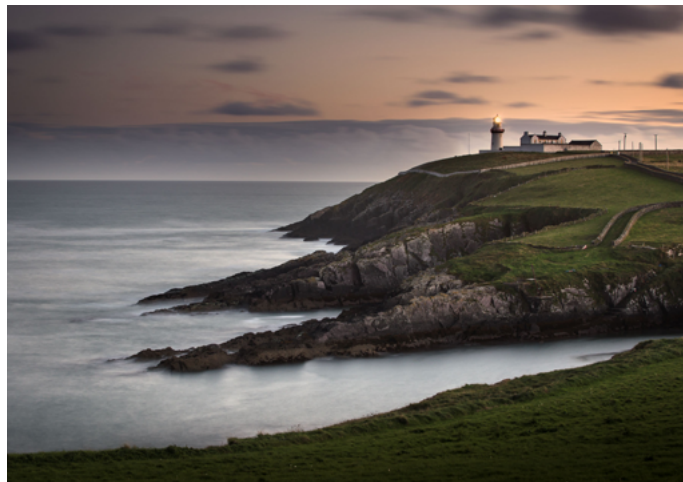
Galley Head Lighthouse, Rosscarbery, County Cork.
